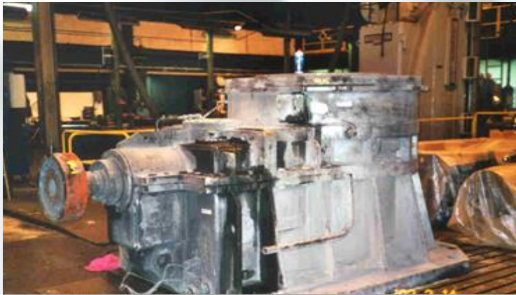
Refurbishment of gearbox for coal crusher
